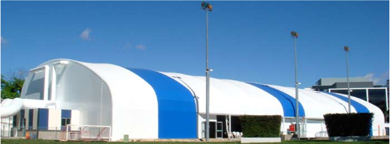
External View - Completed Structure
