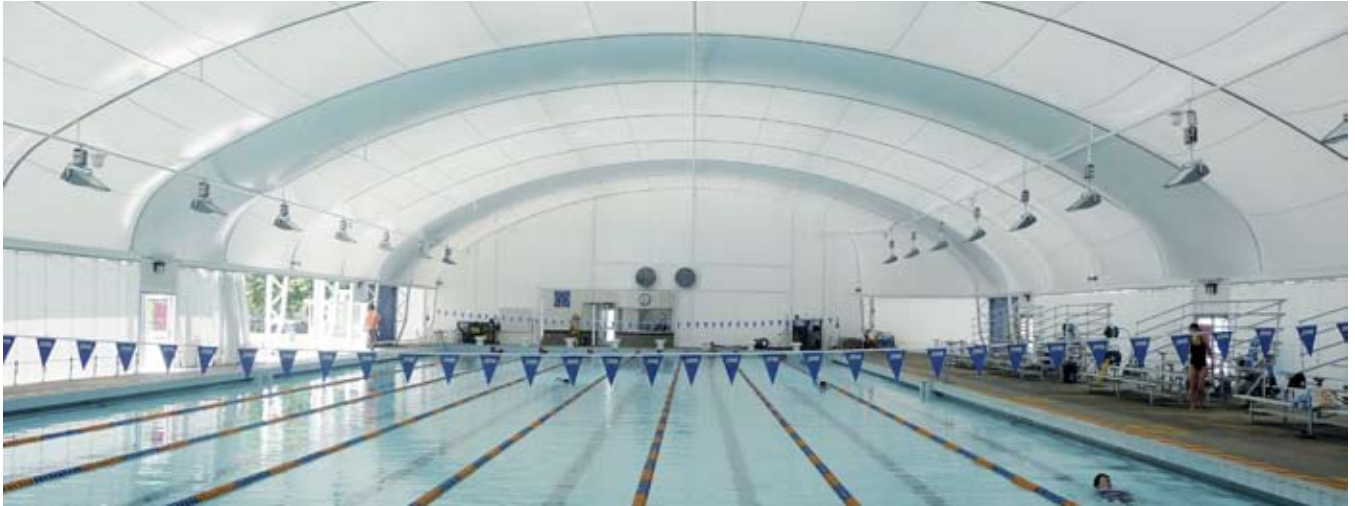
Inside View - Completed Structure
