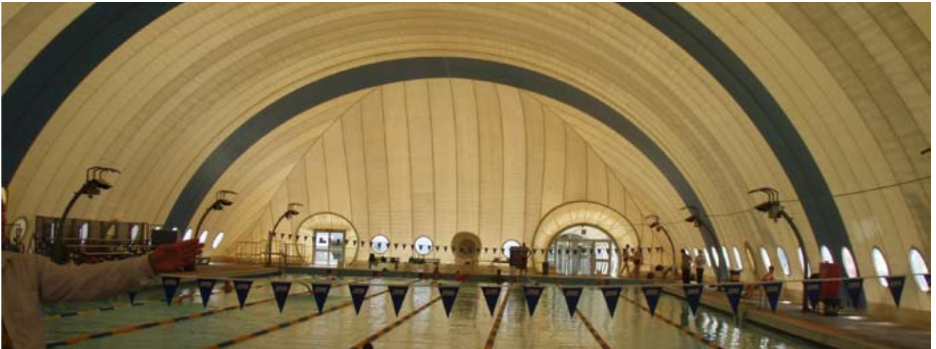
Inside View - Previous Air Supported Membrane
